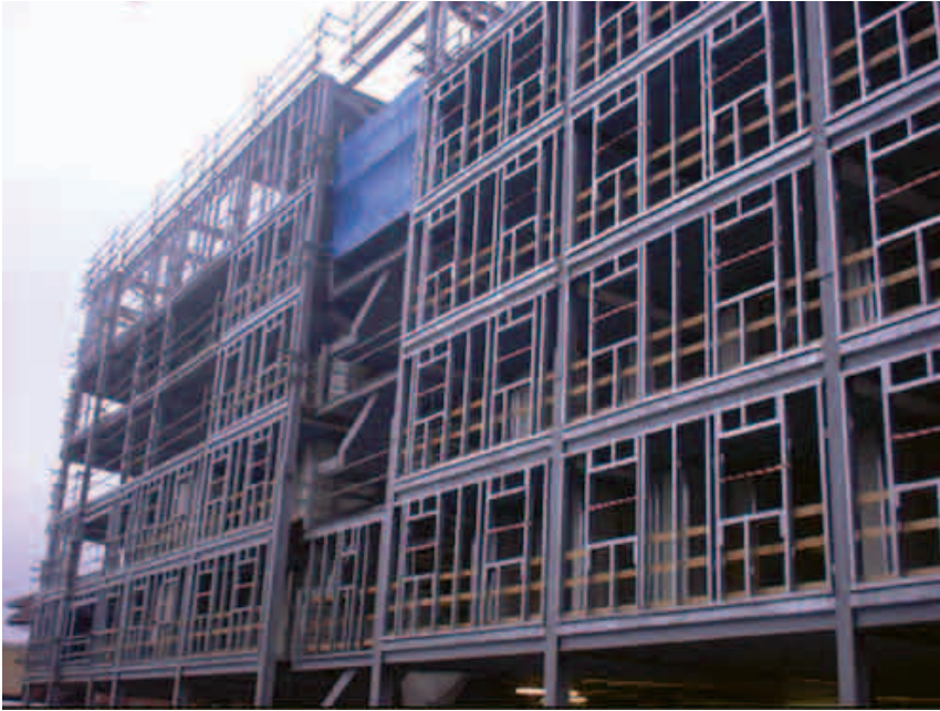
Built with Infill Panels system
